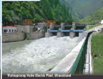
Vishnuprayag Hydro Electric Plant, Uttarakhand
