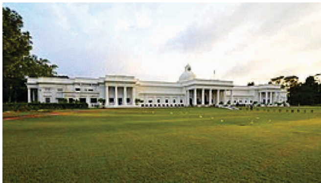
View of IIT Roorkee Admin Building
